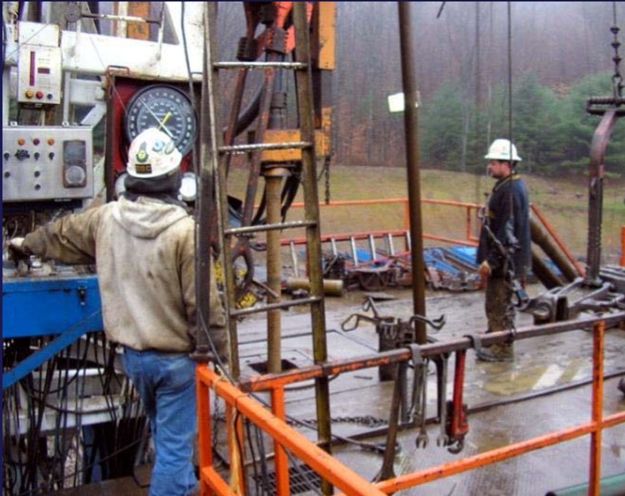
Drilling the Well
